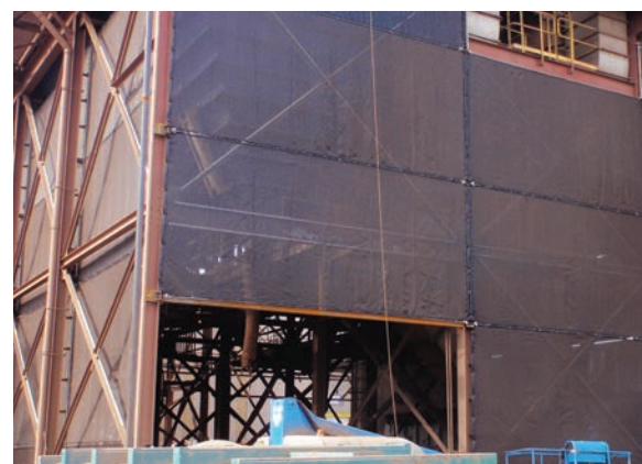
Discharge tower cladding USA 9m (30 ft) x 75m (250 ft)
