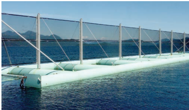
Wind screen on floating breakwater.
