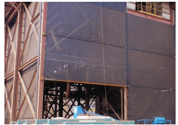
Discharge tower cladding USA 9m (30 ft) x 75m (250 ft)
